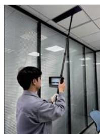
ceiling duct inspection
