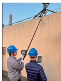
constructure inspection (WIFI real-time image transmission)
